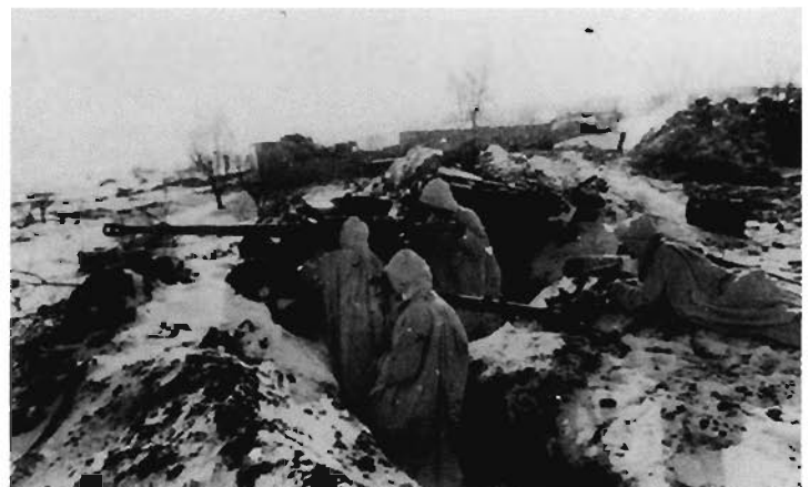
A German Pak 38 anti-tank gun in position with its crew ready to fire. This gun came into service as a replacement for the inadequate 3.7cm Pak 35/36. The Pak 38 basic anti-tank round weighed nearly five pounds and could penetrate the frontal armor of a T-34 at about 500 meters. Later in the war, a shell with a tungsten carbide core was developed which was effective at longer range. (Credit National Archives)
