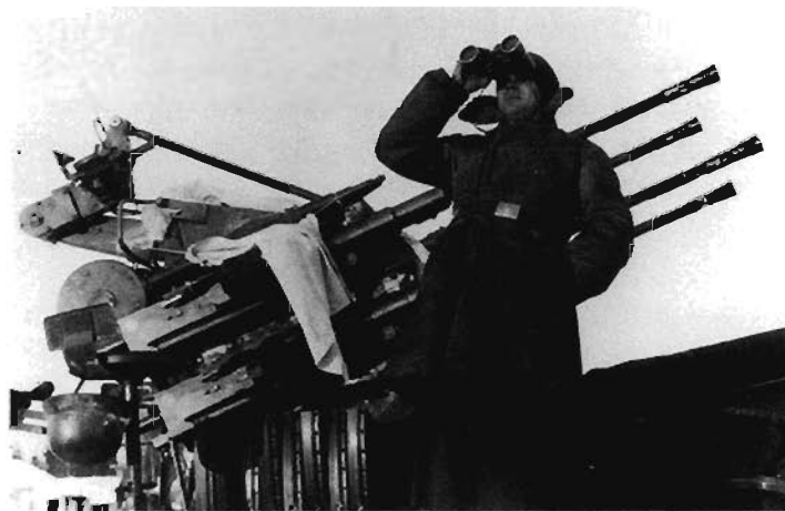
A Flakvierling (four barreled) 2cm anti-aircraft gun of the "Das Reich" Flakabteilung. Stacked beside the base of the gun are spare magazines. The 2cm shells were available in high explosive, incendiary and armor piercing. The Germans used these guns in various configurations, either single guns or the four barreled mount in both anti-aircraft mode or against ground targets. They were extremely effective in both roles. (Courtesy of Mark C. Yerger)
